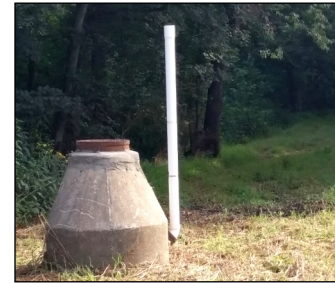
Crews inspect manholes in the town's service areas. Manholes are raised in floodplains, like along Riverwalk.
