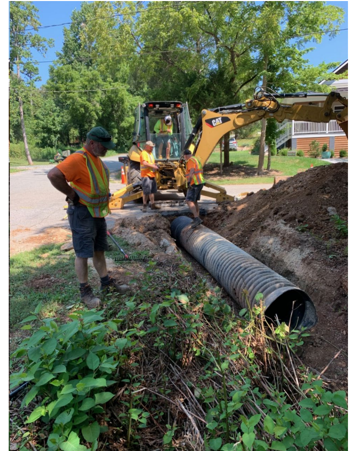
Public Works Staff Completing Stormwater Infrastructure Maintenance
