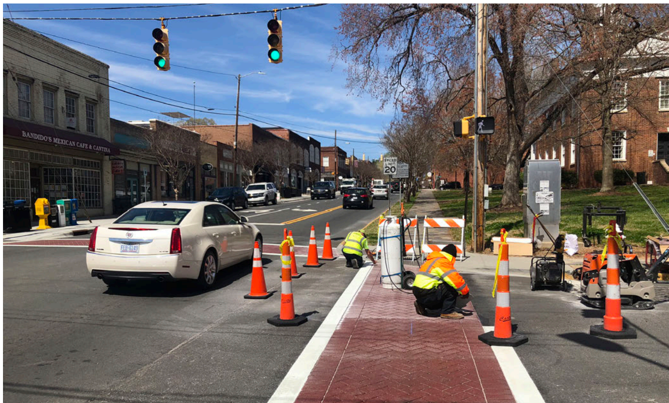
Pedestrian crossing improvements
