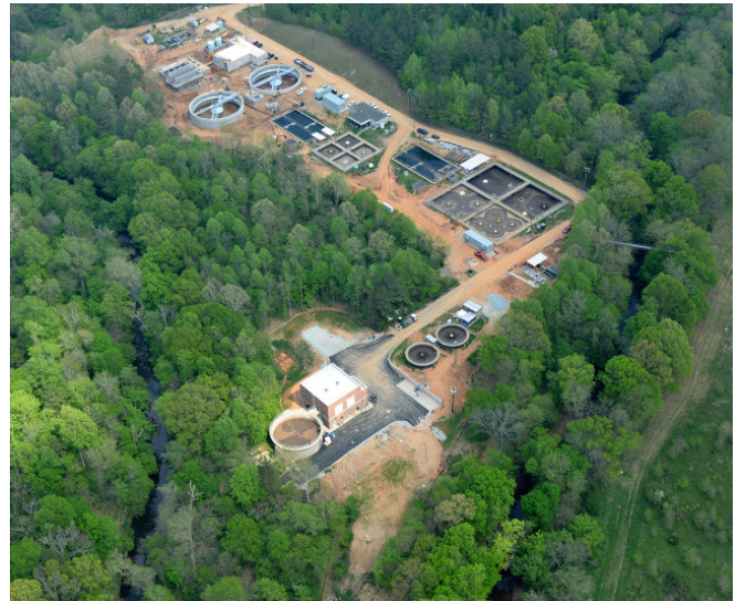
Wastewater treatment plant
