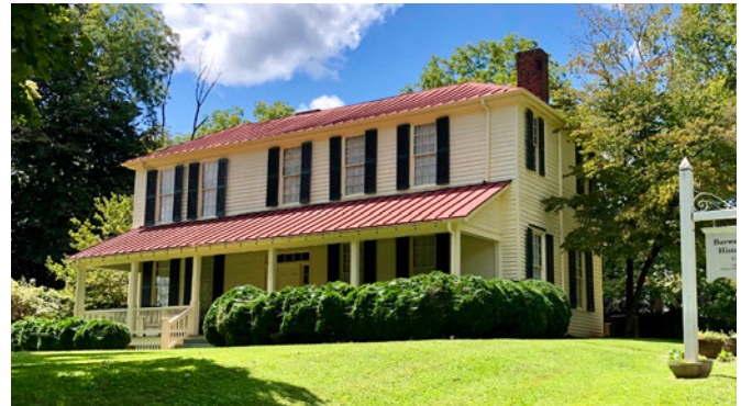
The Burwell School Historic Site is a prominent example of historic architecture within Hillsborough's historic district. The building was built in 1821 and expanded in 1848 to become the location for a girls' school. It was retrofitted to house families through the 19th and 20th centuries.
