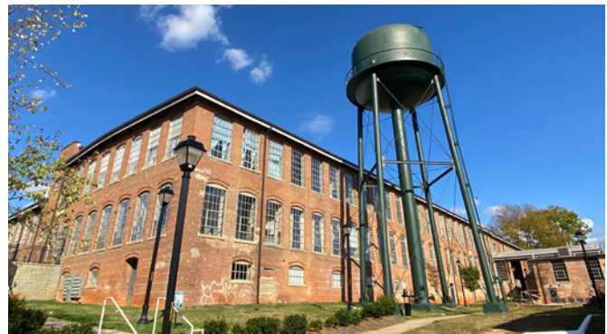
Bellevue Mill — Historic retro-fit apartment complex
