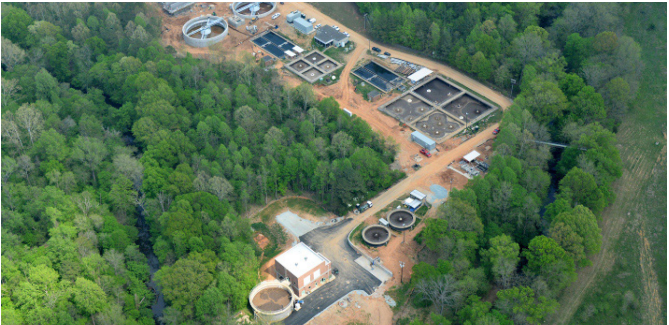
Hillsborough Wastewater Treatment Plant while under an expansion completed in 2014.
