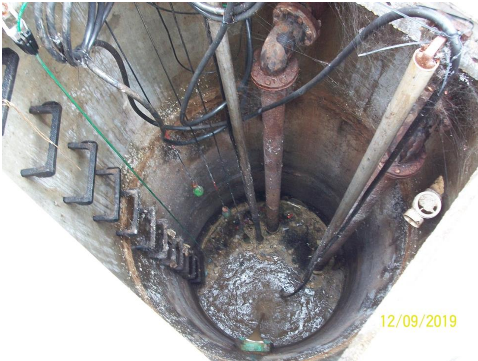
Strouds Creek PS - A newer, "nicer" station. Note little corrosion, room to work. Wet well does have some grease though.
