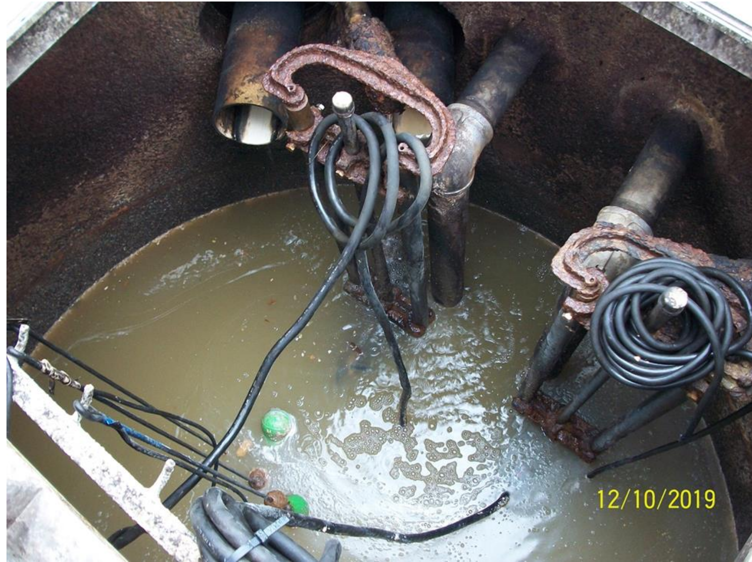
Oakdale Clogged Pump with Rags. 1Timbers PS Wet Well - Note corrosion.
