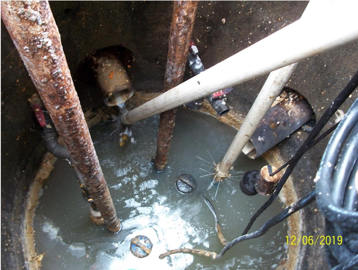
Northside PS - Poor entry holes (gaps), corrosion
