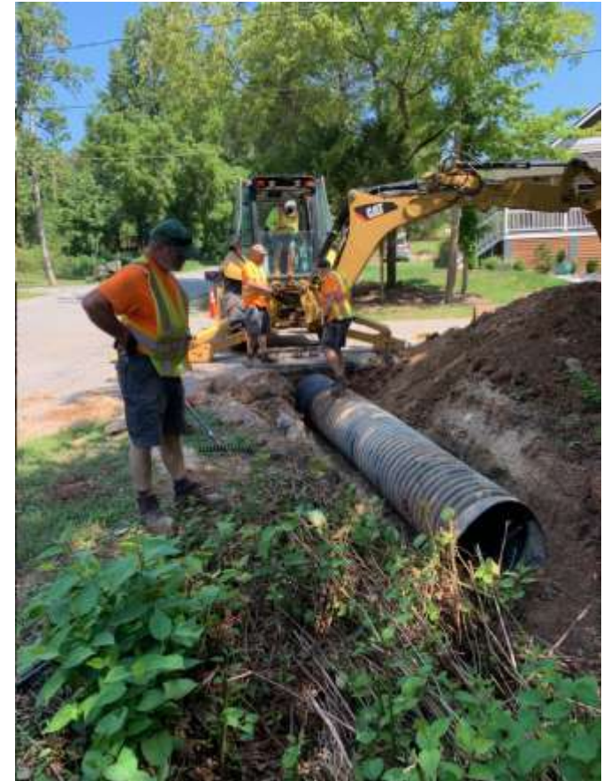
Public Works Staff Completing Stormwater infrastructure Maintenance
