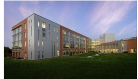
A new patient tower opened in May 2022 at UNC Hospitals Hillsborough Campus.
