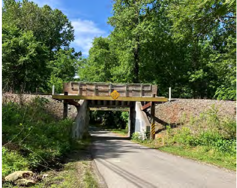
View of North Side of One-Lane Trestle on Exchange Park Lane
