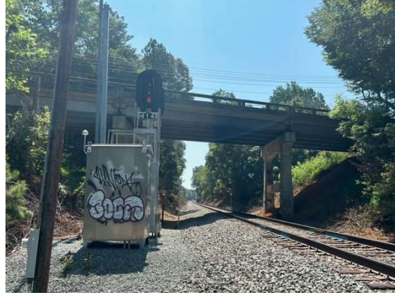
Churton Street bridge over NCRR Operating Corridor
