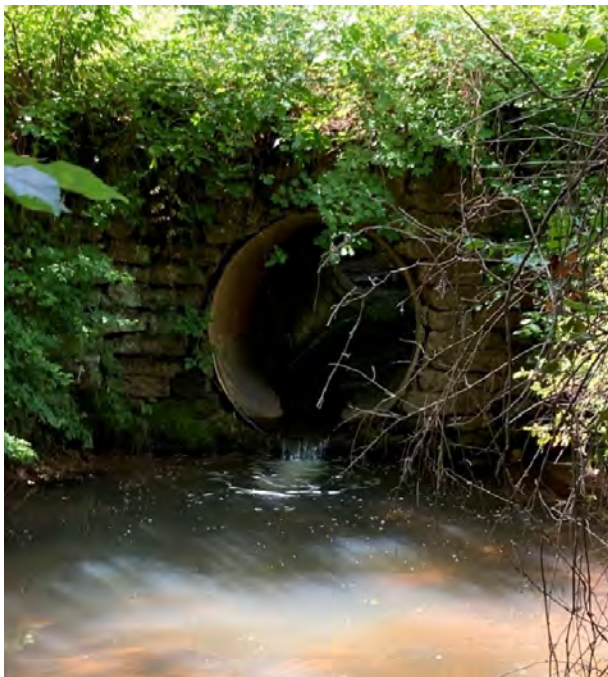
Culvert on Faribault Lane
