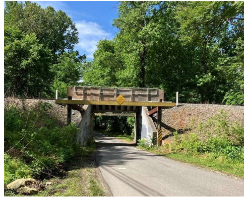
Single lane trestle on Exchange Park Lane
