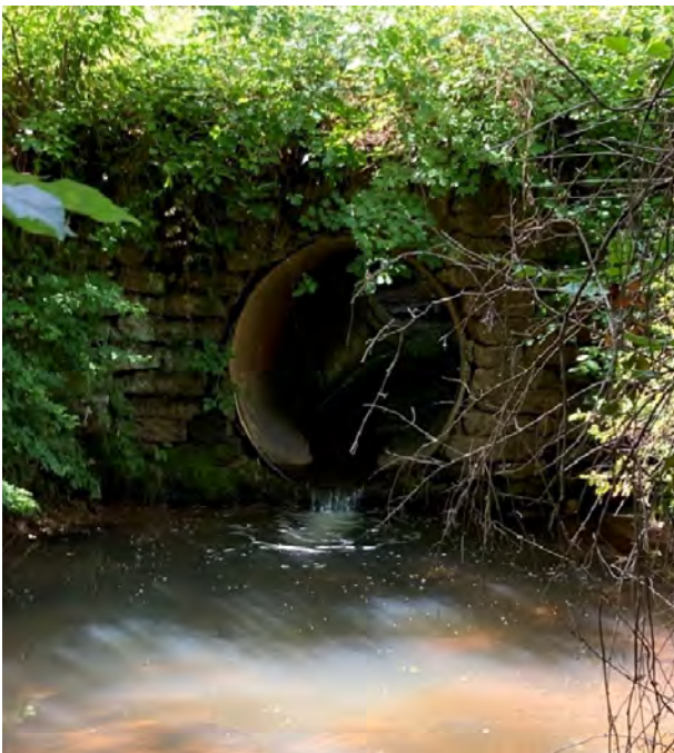
Culvert on Faribault Lane
