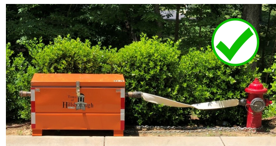
Rented hydrant meter
