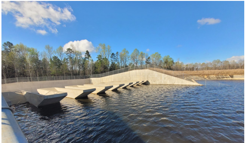
The reservoir's new spillway is designed with notched weirs, also called piano keys because they resemble the instrument's keys.
