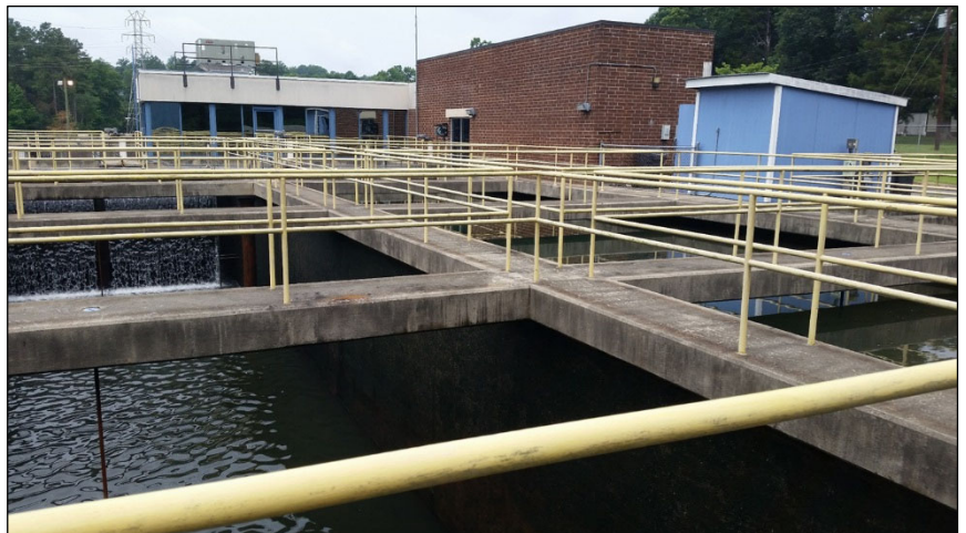
Sedimentation basins at Hillsborough Water Plant
