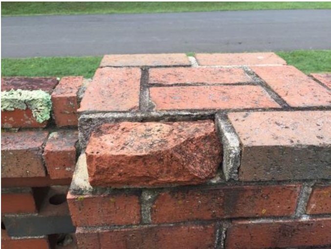
Detail of deteriorating portion of brick wall
