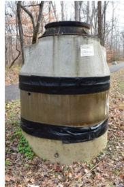
Manholes are much higher than ground level when located in or near a floodplain. The town has more than 2,100 manholes, covering almost 100 miles of sewer system. They range from 3 feet to more than 30 feet deep!
