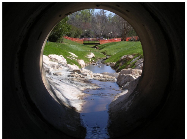
Some stormwater runoff is conveyed through pipes and discharged to a stream. Prior to this section of the creek being restored, stormwater collected in various pipes and then flowed into this pipe under East Margaret Lane, where it flowed into Stillhouse Creek.
