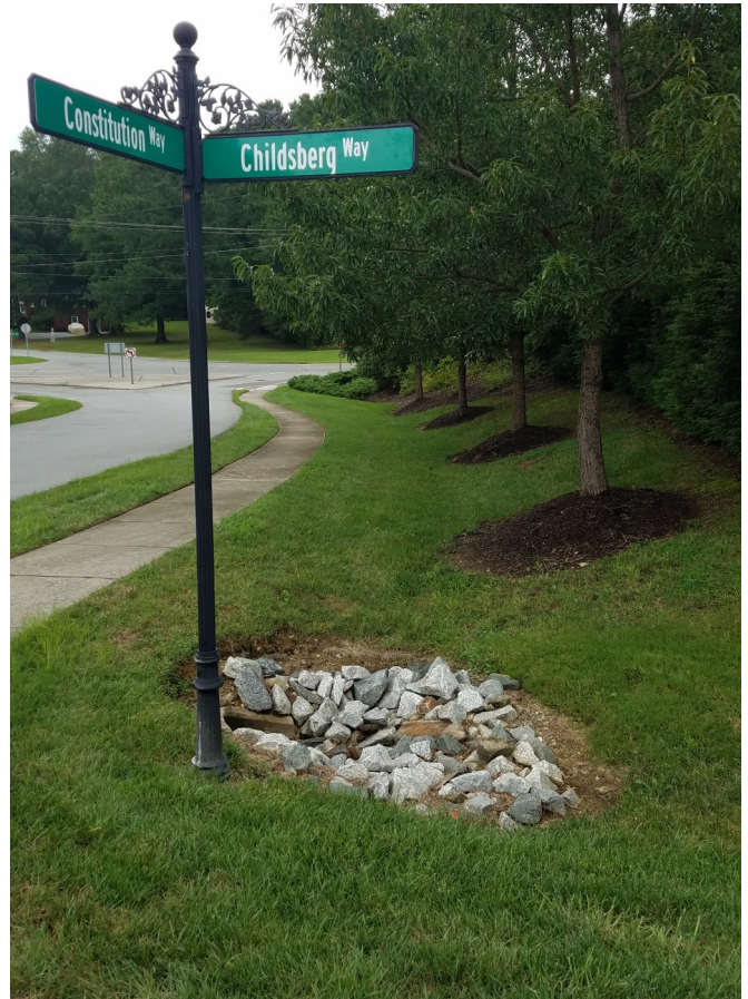
In this well-maintained grass swale in the Kenion Grove neighborhood, water flows into the swale through a pipe under Constitution Way.
