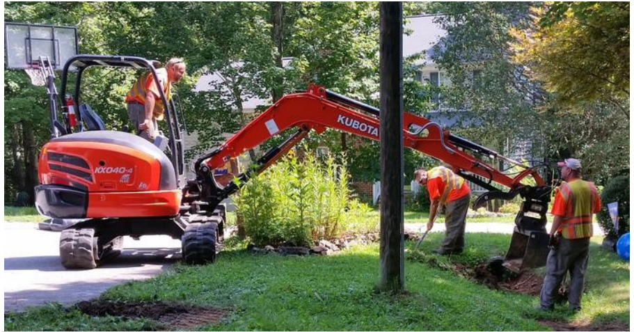
Town Public Works employees operate heavy equipment to dig out a portion of a stormwater drainage system. Hand shovels and rakes also are used to fine-tune the work.
