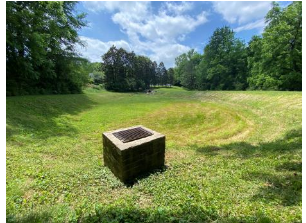
Burke’s Meadow Dry Detention Pond
