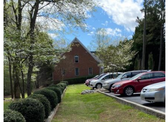
Infiltration Swale at A Step to Health
