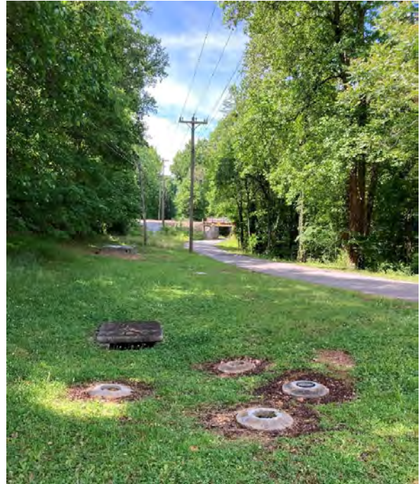
Utilities Next to Exchange Park Lane North of the One-Lane Trestle
