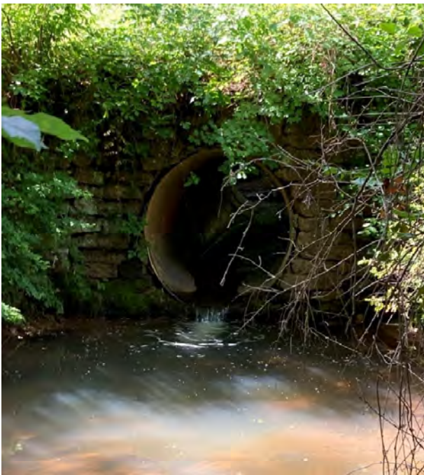
Culvert on Faribault Lane
