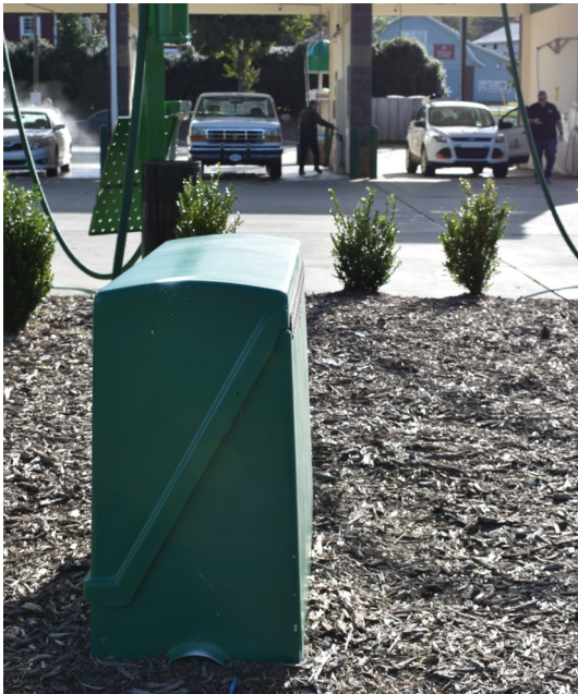
Backflow enclosures like this one (left photo) at a car wash in Hillsborough house backflow prevention devices, which keep contaminants out of the water supply.
