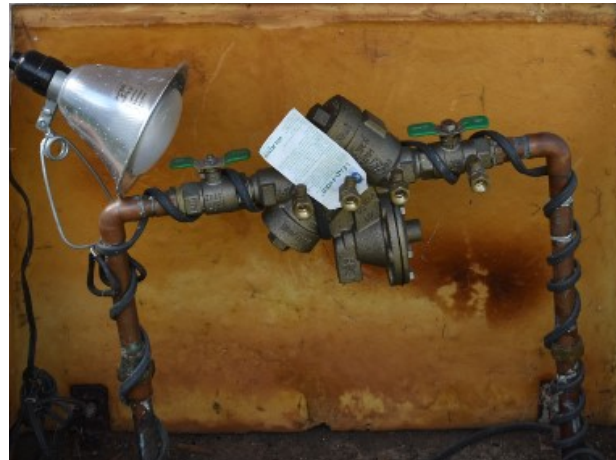
Backflow enclosures like this one (left photo) at a car wash in Hillsborough house backflow prevention devices, which keep contaminants out of the water supply.
