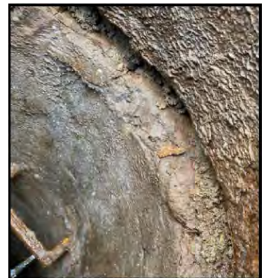
Figure 9: Dirt Intrusion at Frame to Chimney Interface
