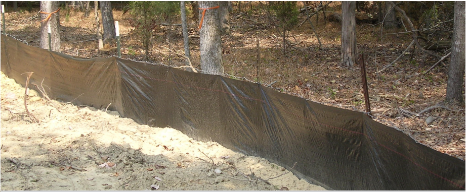
This is a properly installed silt fence. Be sure to trench in the bottom of the fence.
