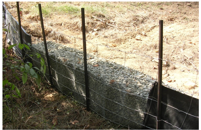
This is a proper silt fence outlet. Be sure to use clean No. 57 stone.
