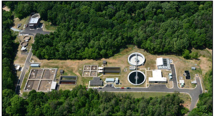
Hillsborough Wastewater Treatment Plant following upgrade in 2014
