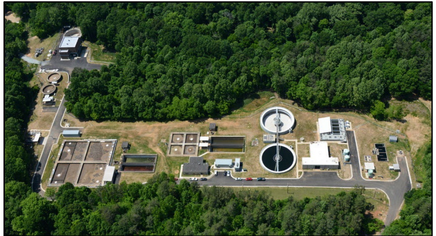
Hillsborough Wastewater Treatment Plant following upgrade in 2014
