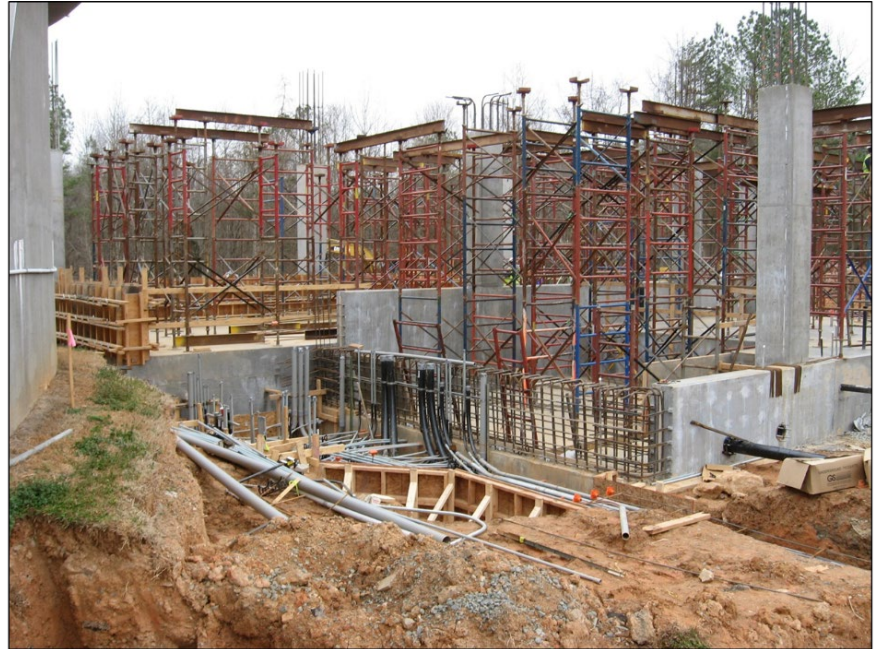
Construction in 2012 to upgrade the Hillsborough Wastewater Treatment Plant
