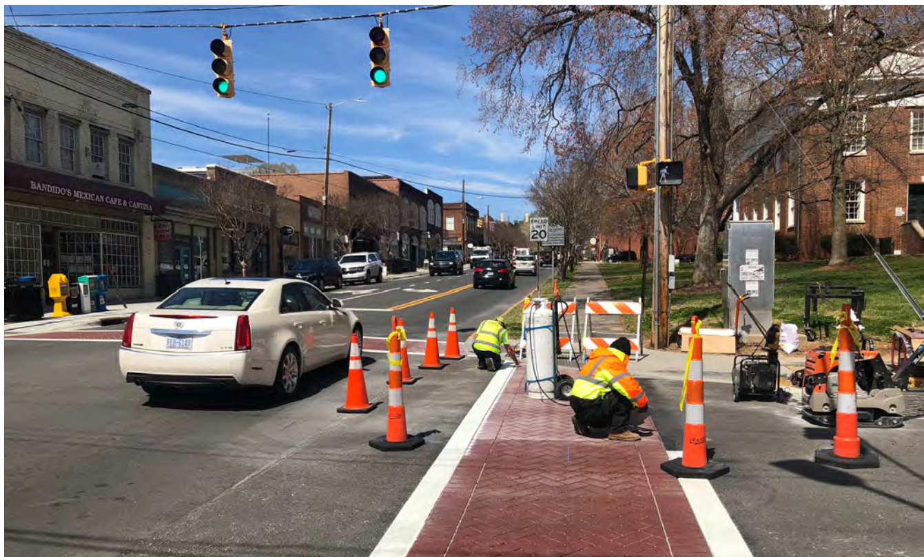
Pedestrian crossing improvements
