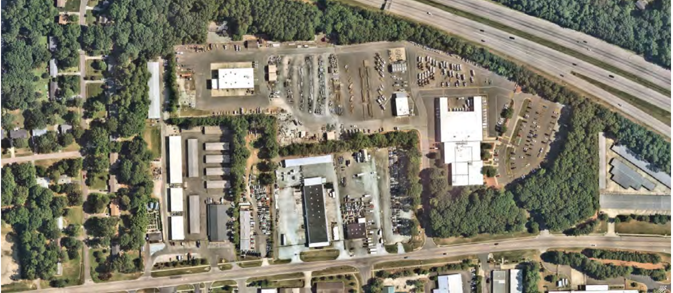
Duke Energy Distribution Center for Hillsborough, Chapel Hill and Durham area
