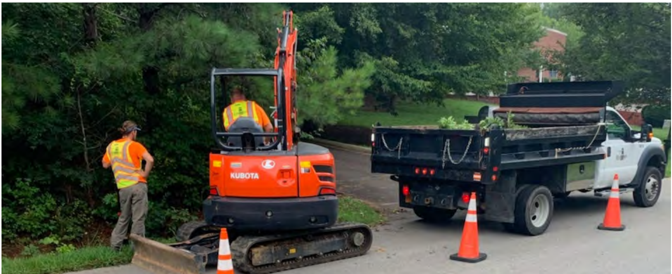
Public works staff conducting maintenance of stormwater ditches.
