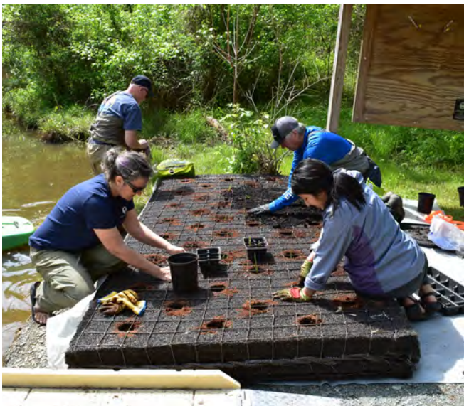
Planting and placing floating wetlands.
