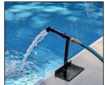
No touching! An air gap keeps the water supply physically separated from a potentially contaminated body of water.
